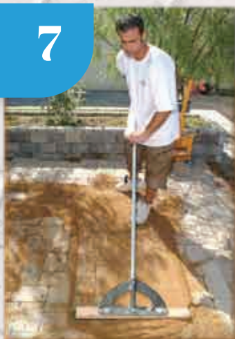
7 Sweep Finishing Sand into Joints
