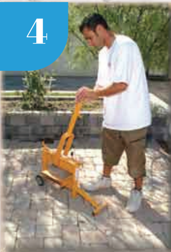
4 Cut Pavers for Edges
