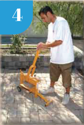
Cut Pavers for Edges
