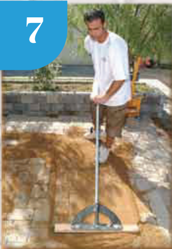
Sweep Finishing Sand into Joints
